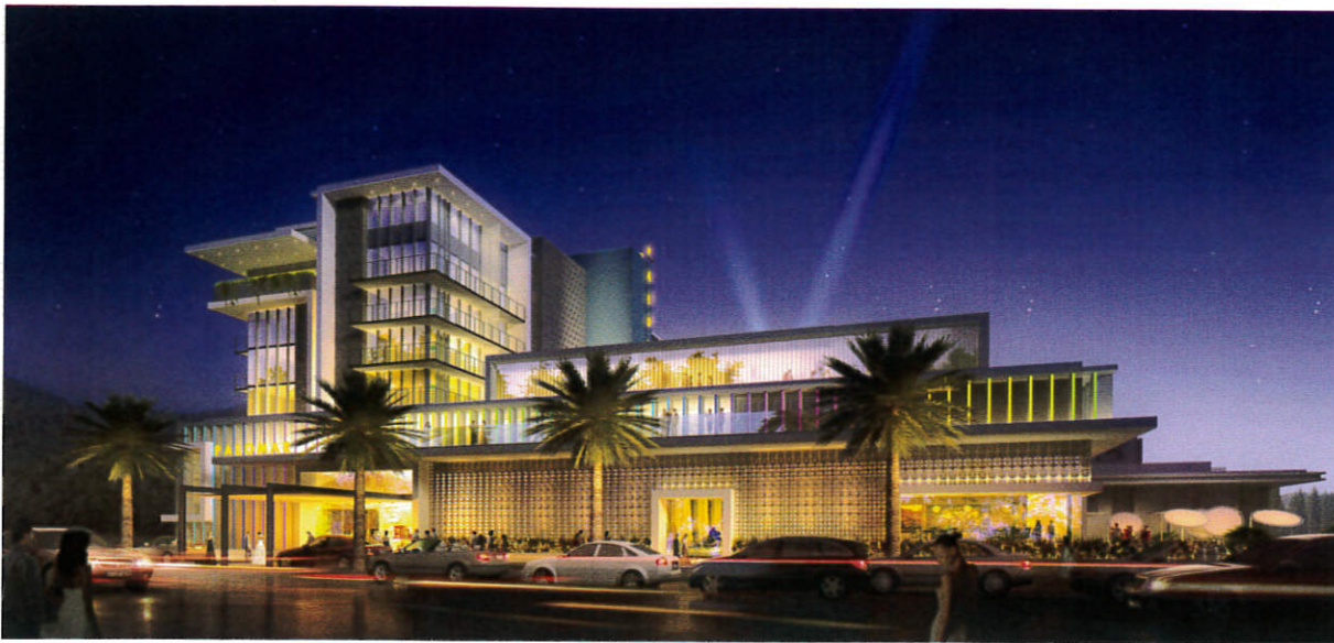
Left: The Palomar, a Kimpton Hotel. Below left to right: Demolition of the old Desert Fashion Plaza. The Hard Rock Hotel under construction.
